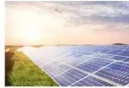
Energy Storage System
